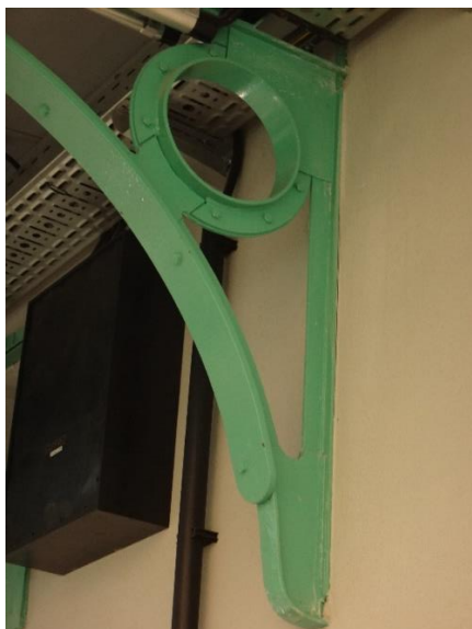
Fig. 11: Detail of the steel structure with bolted-in reinforcing elements Christian Berg 26.09.2020.
