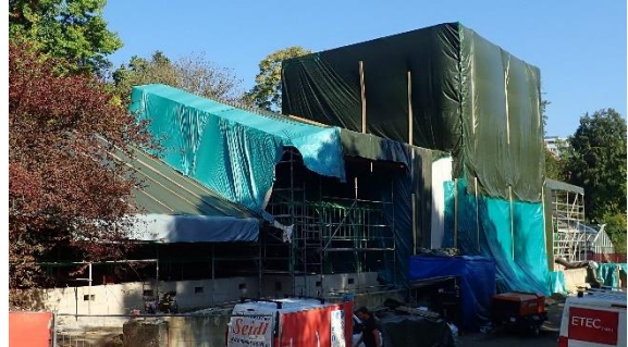
Fig. 8: Enclosure of the building to protect against emissions. Christian Berg 15.09.2020.
