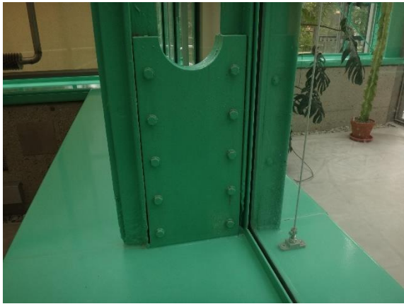
Fig. 10: Detail of the steel structure with screwed-in reinforcing element Christian Berg 29.09.2020
