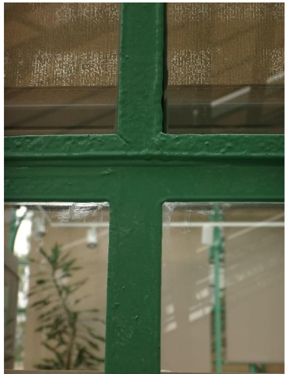
Fig. 9: Detail of the steel structure, above the historical steel, below the renewed steel Christian Berg 29.09.2020.
