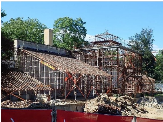
Fig. 7: The steel structure is jacked up. Christian Berg 22.06.2020
